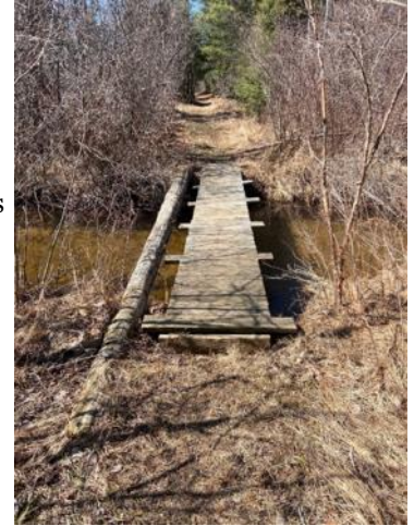
Footbridge on Lossie Road Nature Trail
